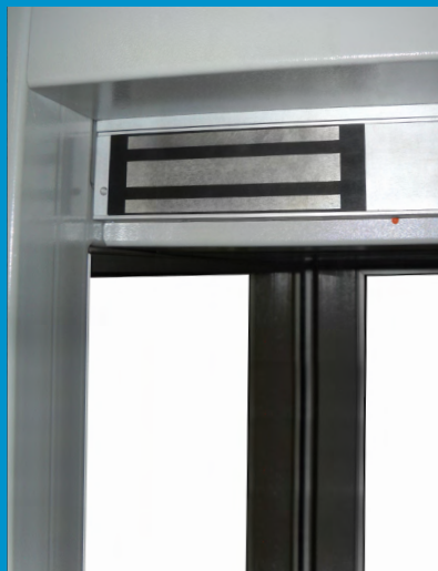
RECESSED 500KG MONITORED MAGNETIC LOCK
